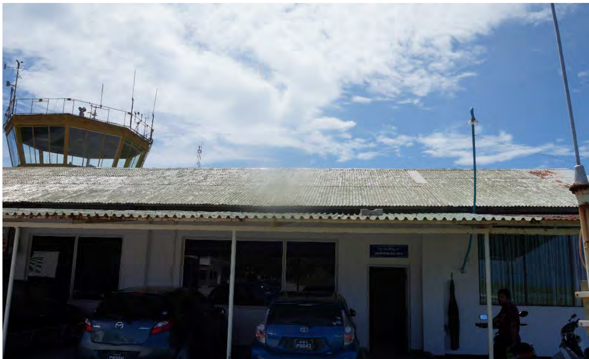
Figure 15: Roof of MET office building
