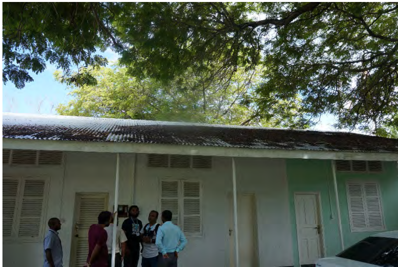
Figure 13: Roof of MET office accommodation unit
