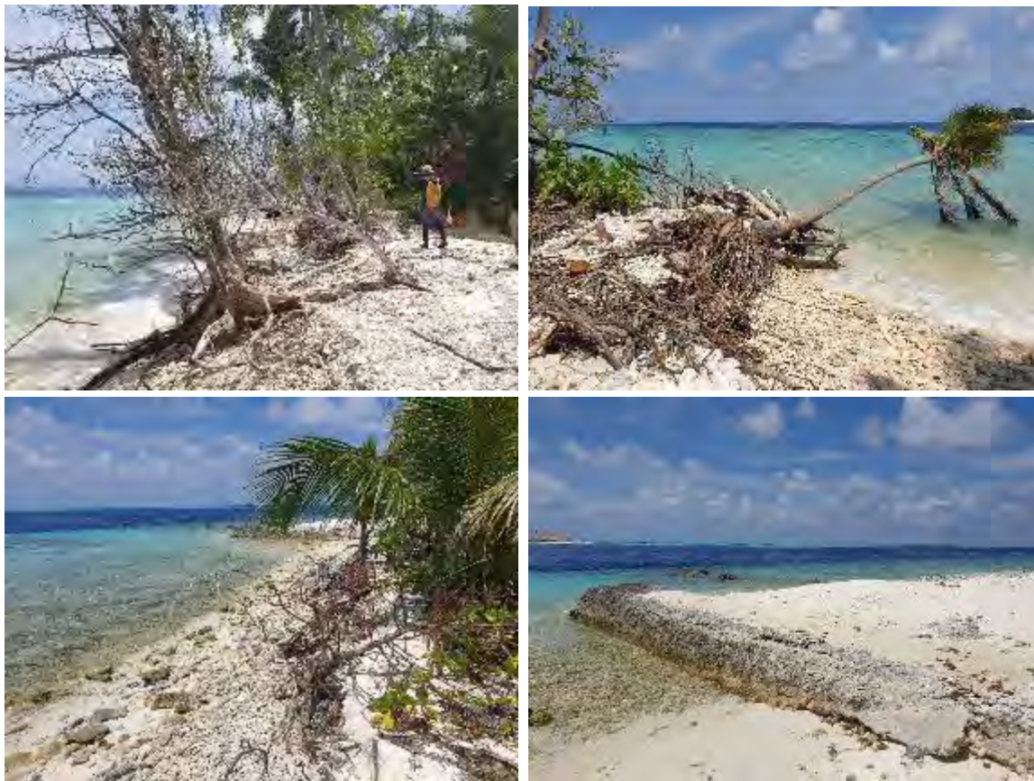
Figure 17. Images of shoreline erosion and (bottom right) the beach protection structures
