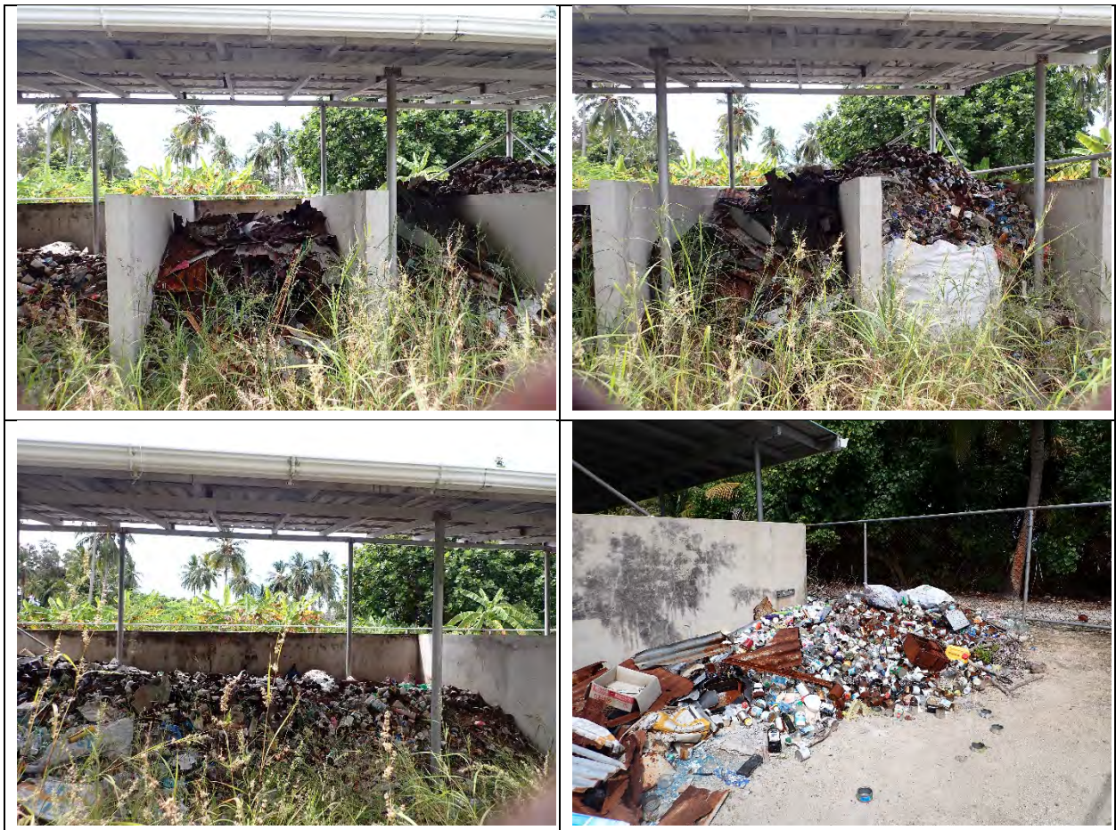
Figure 10. Condition of the existing waste management centre at present
