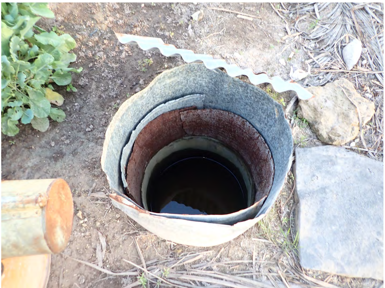
Figure 11. Soil condition at IWRMC site
