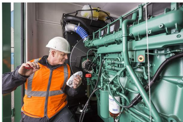
The oil and filter must also be changed at acclimated time intervals. Check with the engine manufacturer for procedures for draining the oil and replacing the oil filter and their disposal is to be done appropriately to avoid environmental damage or liability.
