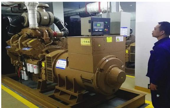
During the running of the diesel generator, the exhaust system, fuel system, DC electrical system and engine require close monitoring for any leaks that can cause hazardous occurrences. As with any internal combustion engine, proper maintenance is essential. Diesels are no exception, and the most important maintenance is oil changes at every 100 hours of operation for a long and trouble-free life assurance.
