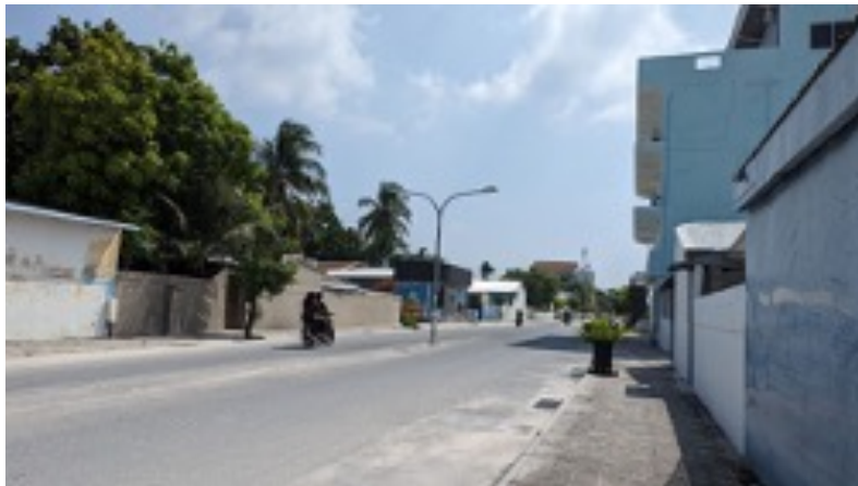
Figure 3: Phase 1 road in Kulhudhuffushi City
