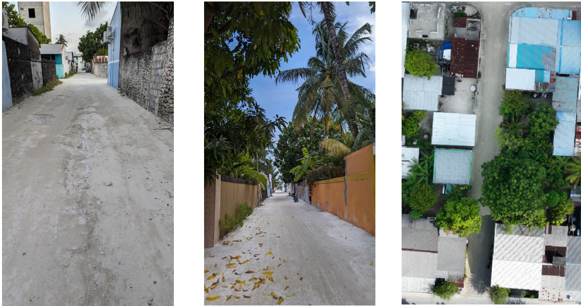
Figure 14: Sample roads in F1 (left), F2 (centre) and F5 (right)
