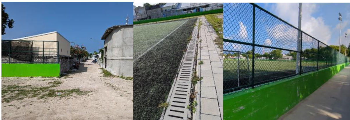
Figure 41: Zigzag Stadium in Kulhudhuffushi, with an aquacell field underneath
