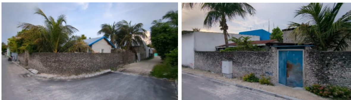
Figure 36: Traditional coral compound walls in Kulhudhuffushi
