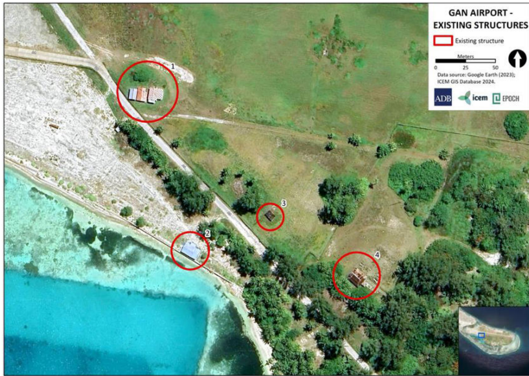
Figure 34: Existing structures south of the runway at Gan
